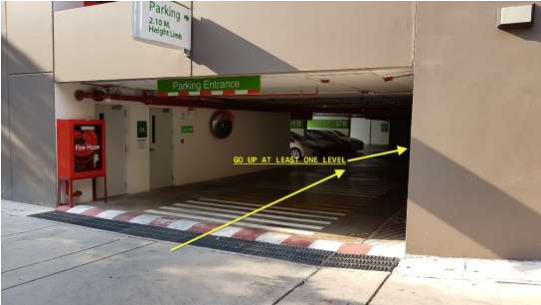
Enter into the Parking Garage and go up at least one level for free parking.
